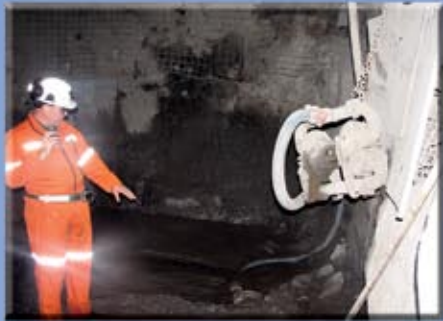
Mud & Muck Pumping
